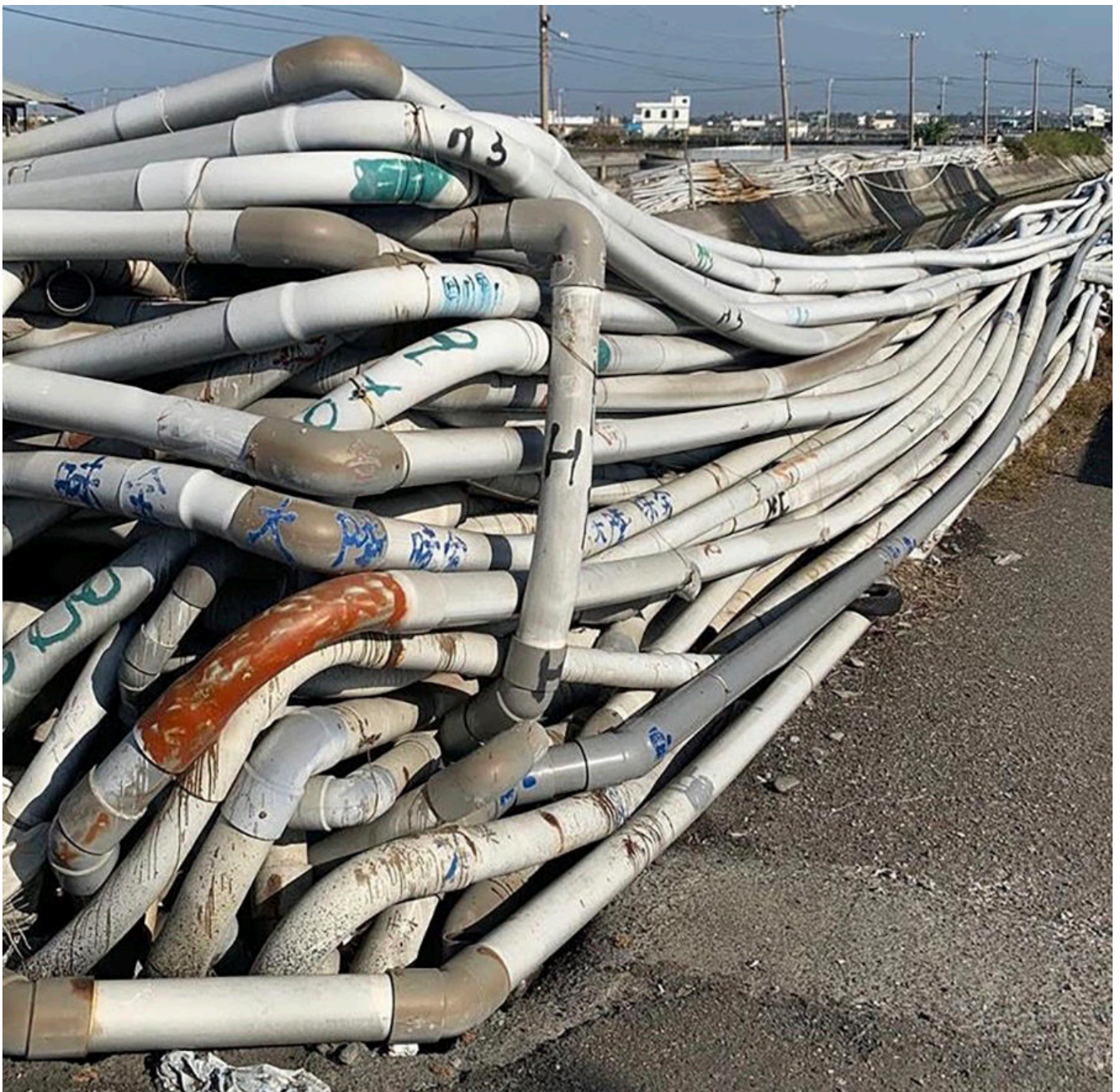
Entangled water pipes pumping groundwater for fish farms in Jiadong County, Taiwan. The sheer volume extracted over decades has led to subsidence all over the region. / Photo by Cooking Sections, 2019.
